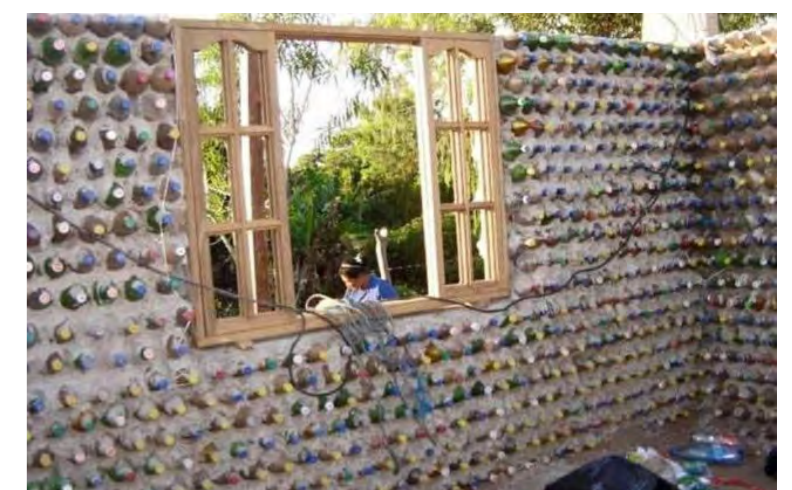
Wasted Waer Bottle as Recycled Constuction Material
