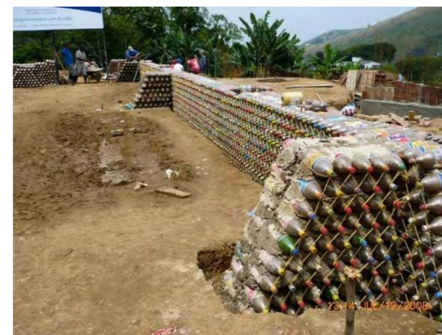
Wasted Waer Bottle as Recycled Constuction Material
